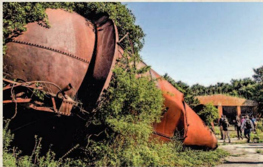
A 2019 file photo shows a toppled water tower lying next to the water tower maintenance shop and firehouse on Gould Island, among the relics of the U.S. Navy's torpedo testing site on the island during World War II. DAVID DELPOIO/THE PROVIDENCE JOURNAL
